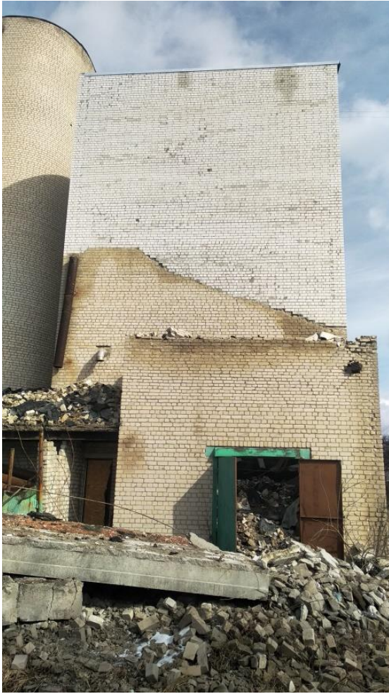
Fig.6. Restored walls and roof of destroyed building
