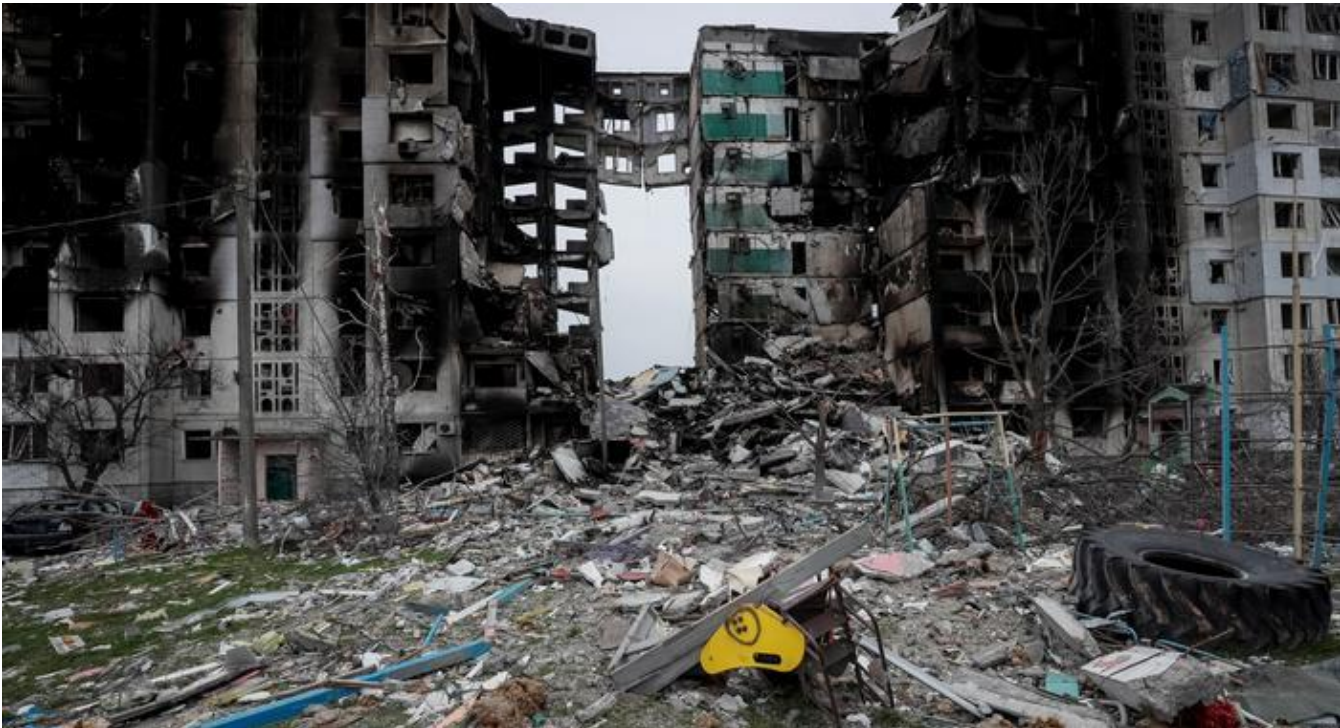
Destroyed residential building in Borodyanka, Kyiv region
